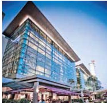
Bangsar Shopping Centre Bangsar
